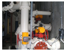
A NEW ADDITION TO OUR WATER TREATMENT PLANT IN 2010 WAS THE CONSTRUCTION OF THIS 1800 GPM GRANULAR ACTIVATED AUTOMATED WATER FILTER
